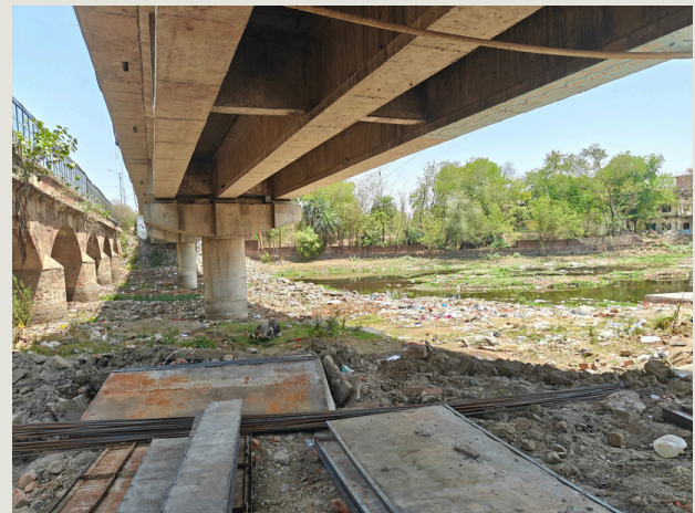
Ongoing efforts towards interception and diversion of drains discharging into the Pahuj River
